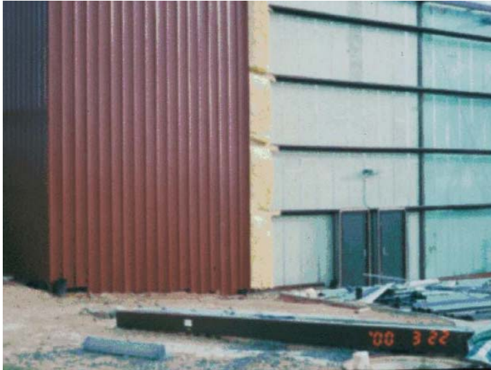
Poor wall insulation detail
