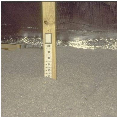
Ruler shows depth of installed blown-in insulation. Typical blown-in insulation has an R-value of around R-3.2 per inch. 12 to 14 inches of blown-in insulation is typical to achieve R-38.
