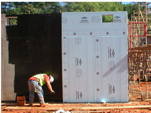
Installation of a waterproof coating installed under continuous insulation on a concrete wall.
