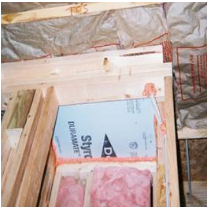
CORRECT: Well-sealed chase
