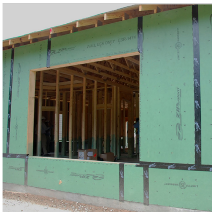
Sheathing seams properly sealed
