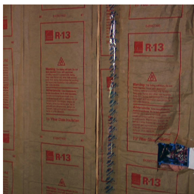
CORRECT: Full coverage/no compression
