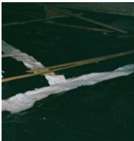
Sealed and overlapped seams
