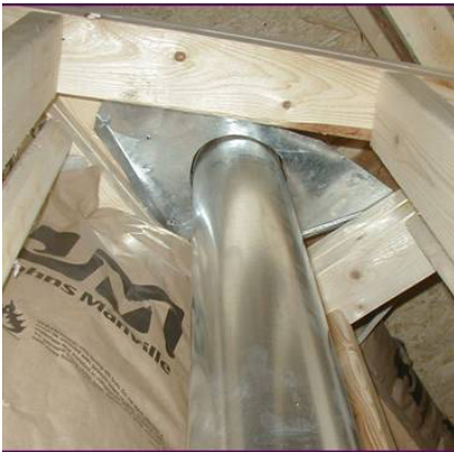
INCORRECT: Improperly capped chase
