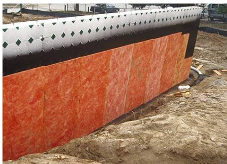
Insulated concrete form exceeds code by providing continuous insulation on interior and exterior of foundation.
