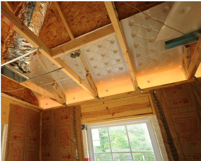
Baffles (pre-insulation) extended over top-plate
