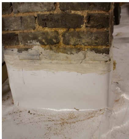
Sealed and applied 6" up wall
