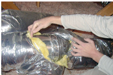
CORRECT: Mastic-sealed Joints
