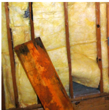
INCORRECT: Unfilled cavity
