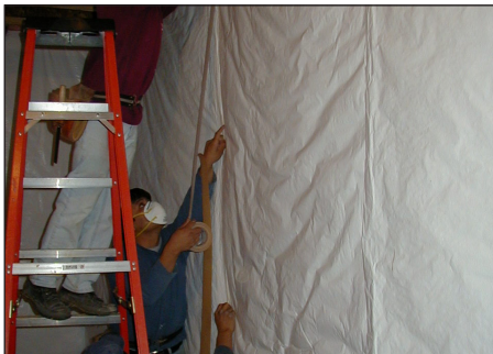
Insulation installed in full contact with wall.
