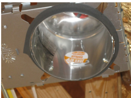
CORRECT: IC-rated and air-tight
