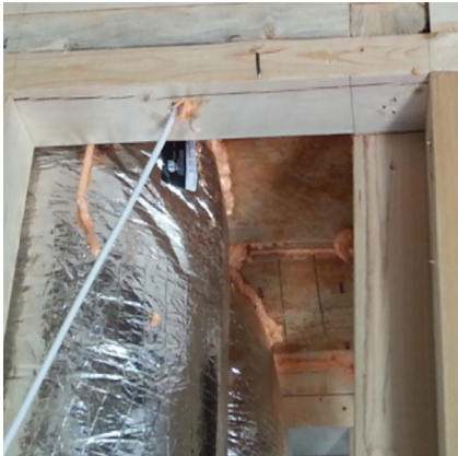
CORRECT: Capped chase properly sealed
