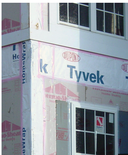
CORRECT: Tape seams in house wrap
