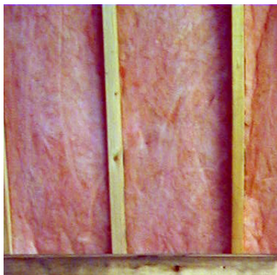
CORRECT: Batt in wood-framed cavity
