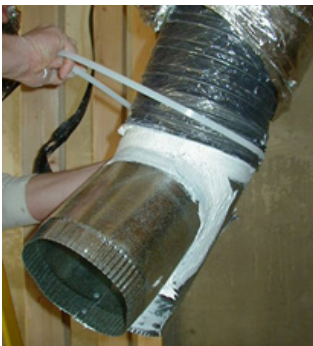
CORRECT: Mastic-sealed Joints
