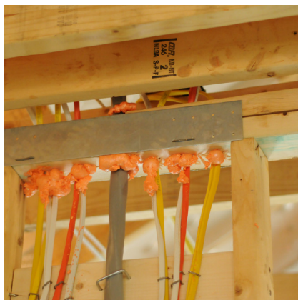
CORRECT: Air-sealed utility penetrations
