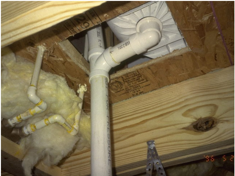
INCORRECT: Drain penetration open
