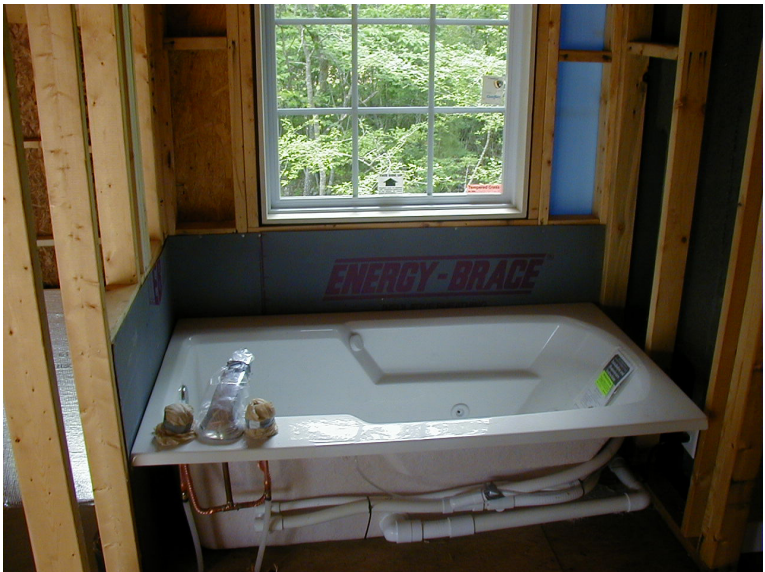
CORRECT: Air barrier and insulation behind tub
