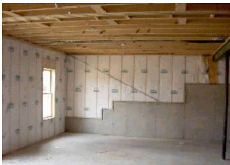
INCORRECT (CZ3): Insulation not on concrete portion of basement wall.
