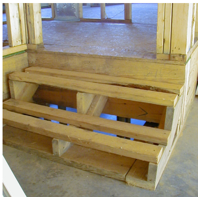
INCORRECT: Air bypass behind stairs
