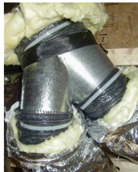
INCORRECT: UL-181 Tape without Mastic
