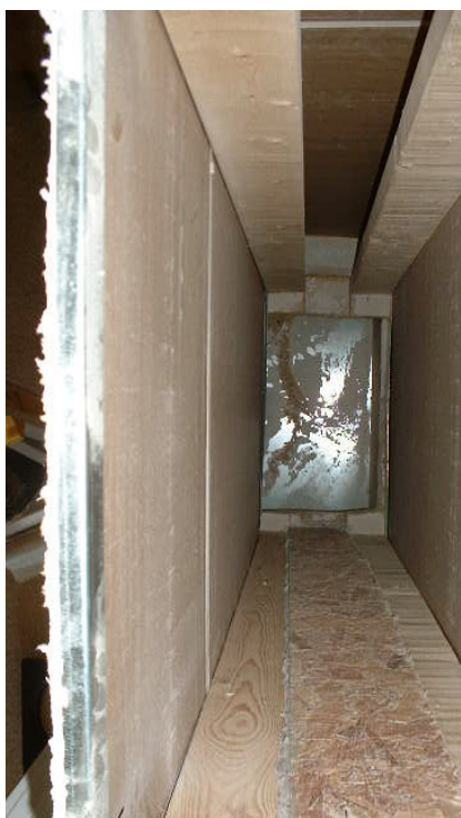
INCORRECT: Unlined cavity as plenum
