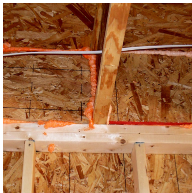
CORRECT: Joist cavities blocked
