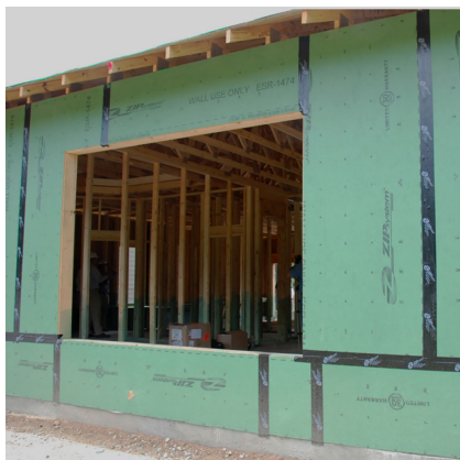
Sheathing seams properly sealed
