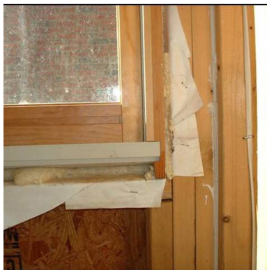
Air-sealing with spray foam
