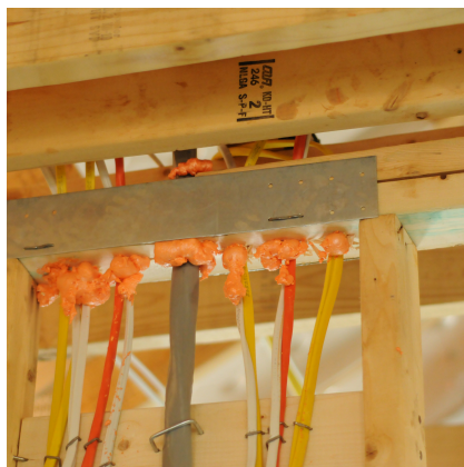
CORRECT: Air-sealed utility penetrations
