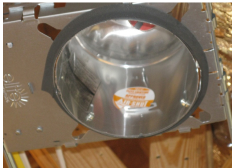
CORRECT: IC-rated and air-tight
