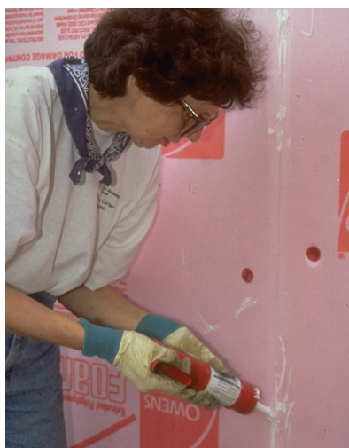
CORRECT: Sealing exterior sheathing
