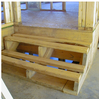
INCORRECT: Air bypass behind stairs
