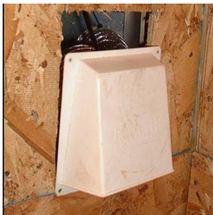
INCORRECT: Unsealed sheathing penetration
