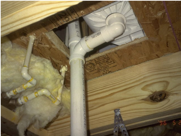
INCORRECT: Drain penetration open
