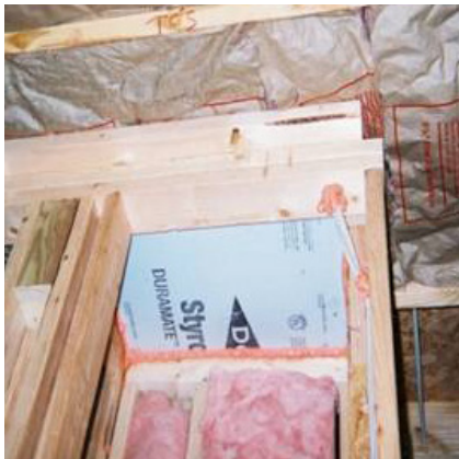
CORRECT: Well-sealed chase
