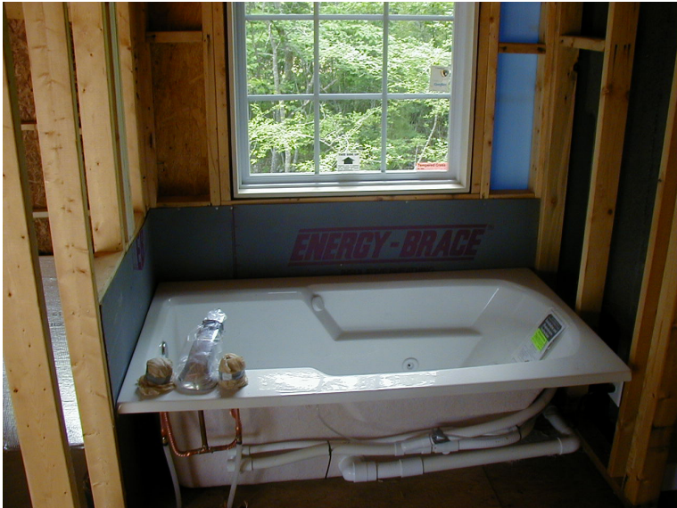
CORRECT: Air barrier and insulation behind tub
