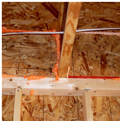
CORRECT: Joist cavities blocked
