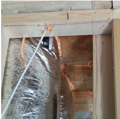
CORRECT: Capped chase properly sealed
