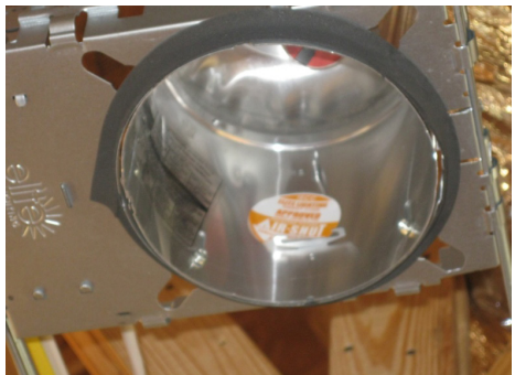
CORRECT: IC-rated and air-tight
