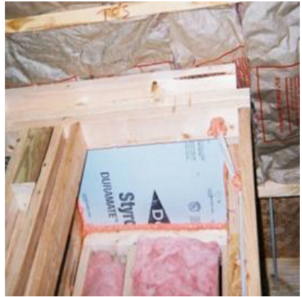
CORRECT: Well-sealed chase
