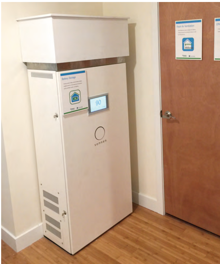
A battery storage system located in a low-income housing rental property for resilient power and cost savings. This installation was supported by Clean Energy Group's Resilient Power Project. Photo: Clean Energy Group
