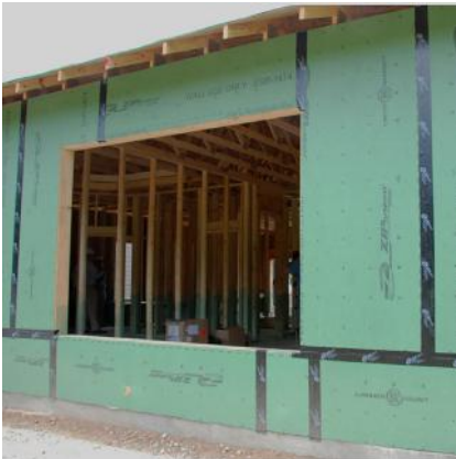
Sheathing seams properly sealed
