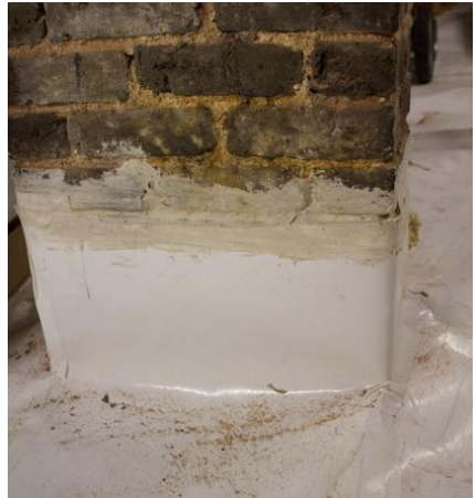
Sealed and applied 6" up wall
