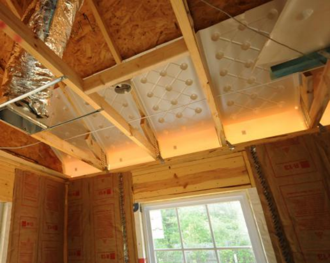
Baffles (pre-insulation) extended over top-plate
