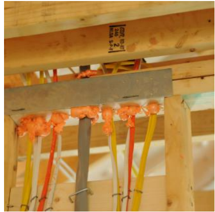
CORRECT: Air-sealed utility penetrations
