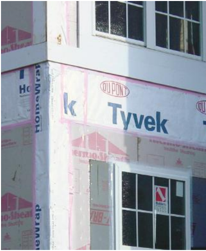
CORRECT: Tape seams in house wrap
