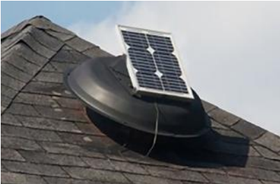
ALLOWED: Solar-powered ventilator
