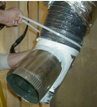
CORRECT: Mastic-sealed Joints
