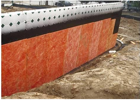
Insulated concrete form exceeds code by providing continuous insulation on interior and exterior of foundation.
