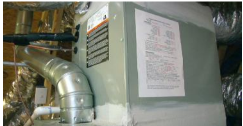
Compliance certificate affixed to electrical panel or main air handler
