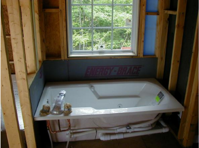
CORRECT: Air barrier and insulation behind tub
