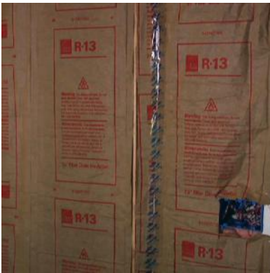
CORRECT: Full coverage/no compression
