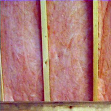
CORRECT: Batt in wood-framed cavity
