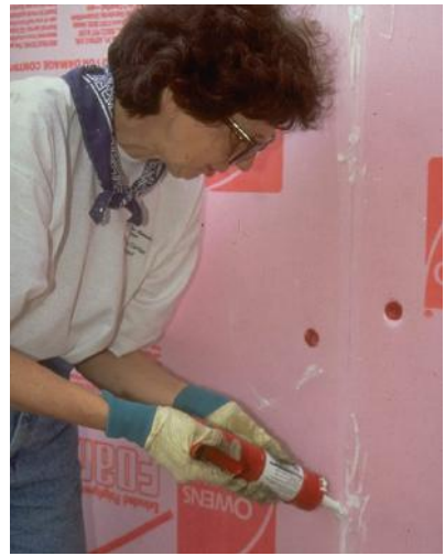
CORRECT: Sealing exterior sheathing
