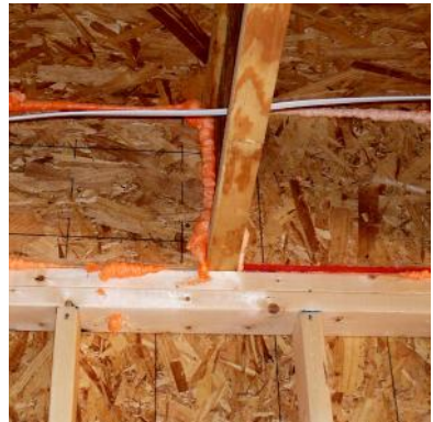
CORRECT: Joist cavities blocked
