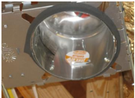
CORRECT: IC-rated and air-tight
