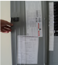
Compliance certificate affixed to electrical panel or main air handler
