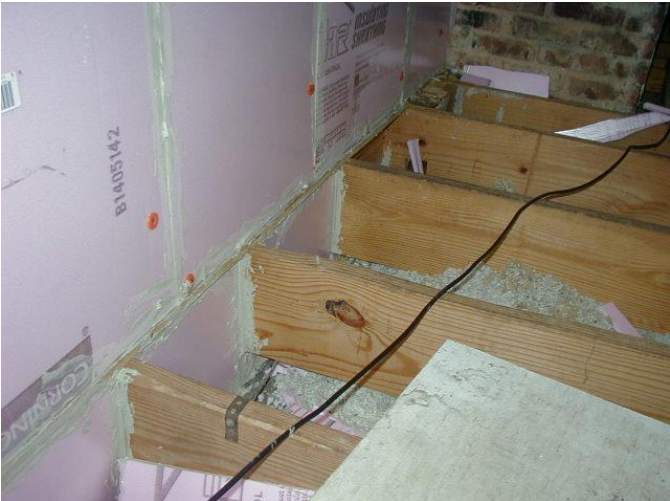
CORRECT: Blocked joist cavity/sealed attic-side air barrier
