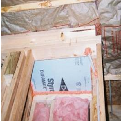
CORRECT: Well-sealed chase
