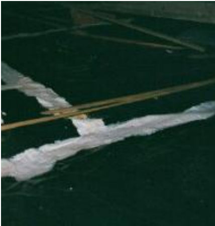
Sealed and overlapped seams
