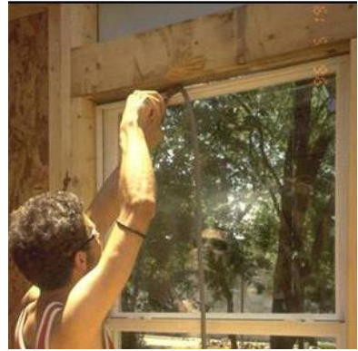
Air-sealing with backer rod
