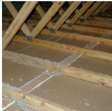
Ceiling drywall sealed to top plate from attic side
