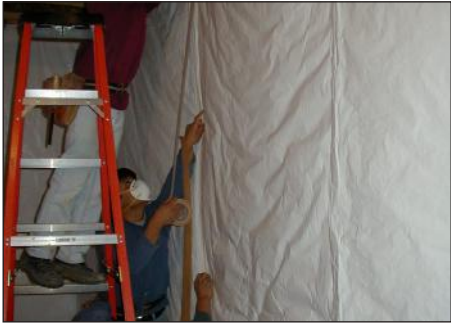
Insulation installed in full contact with wall.
