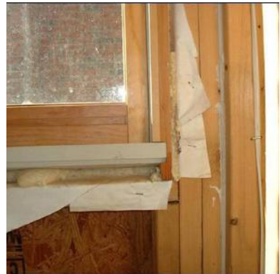
Air-sealing with spray foam
