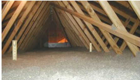
Blown insulation rulers installed 1 per 300 sq. ft. facing attic access
