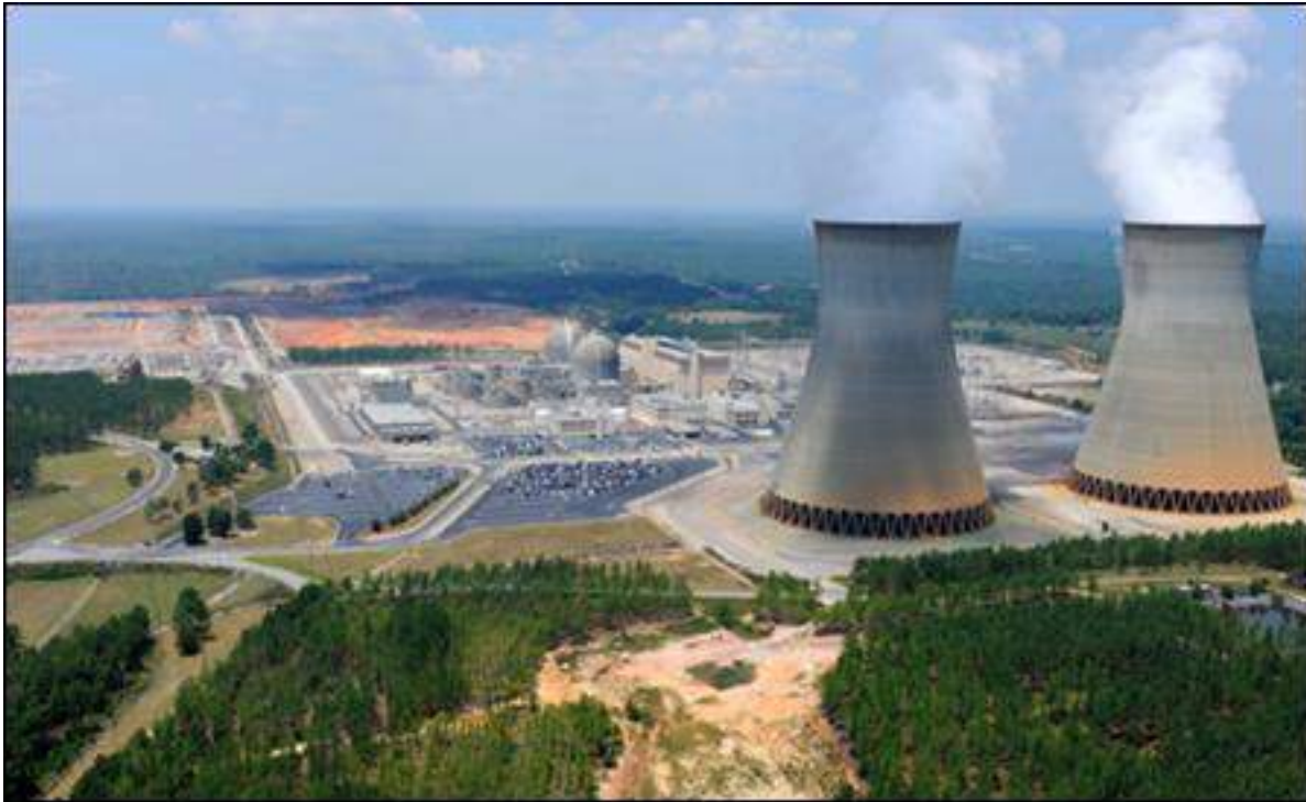
Photo credit: Georgia Power.
