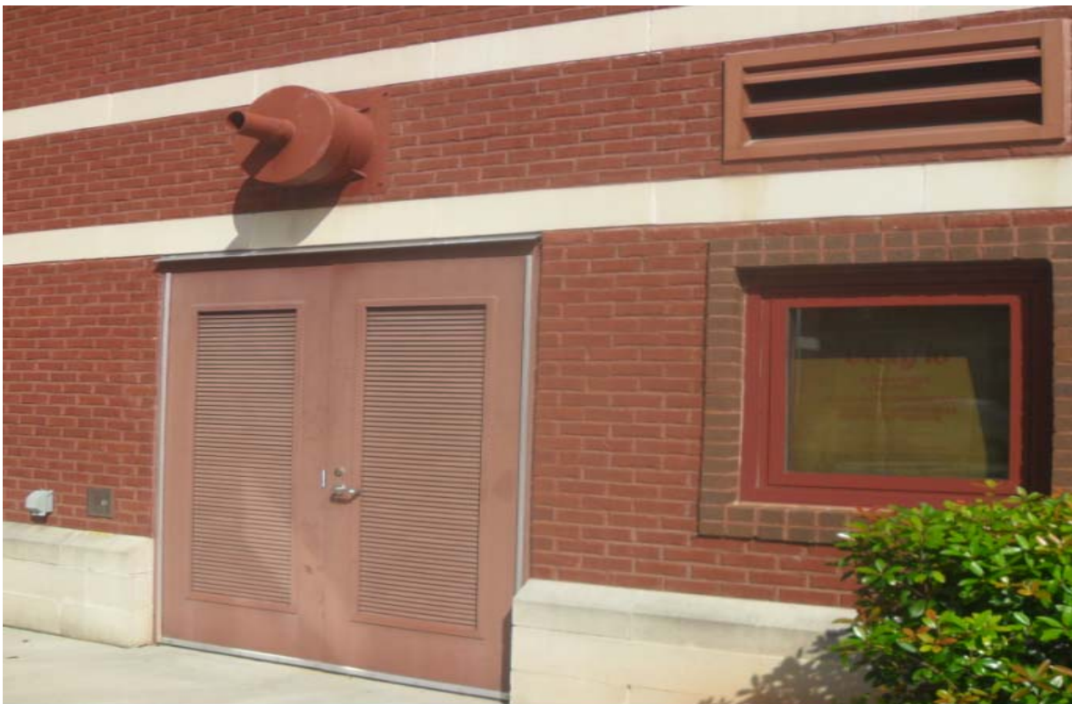
Figure 14: A massive diesel generator resides behind these doors – this space must be carefully air sealed from the rest of the building and confirmed through diagnostic testing. Is this an Outside Air (OA) intake located above the window that is so close to the diesel exhaust? (Fire4) [Barcik photo]
