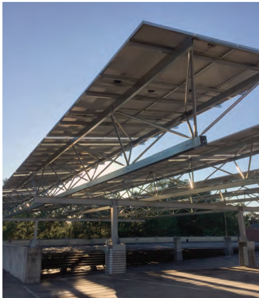
The West Parking array (left) features the innovative QuadPod racking design. The Bradley Observatory array (right) is used by students and faculty as a hands-on teaching tool. Photos courtesy Inman Solar.
