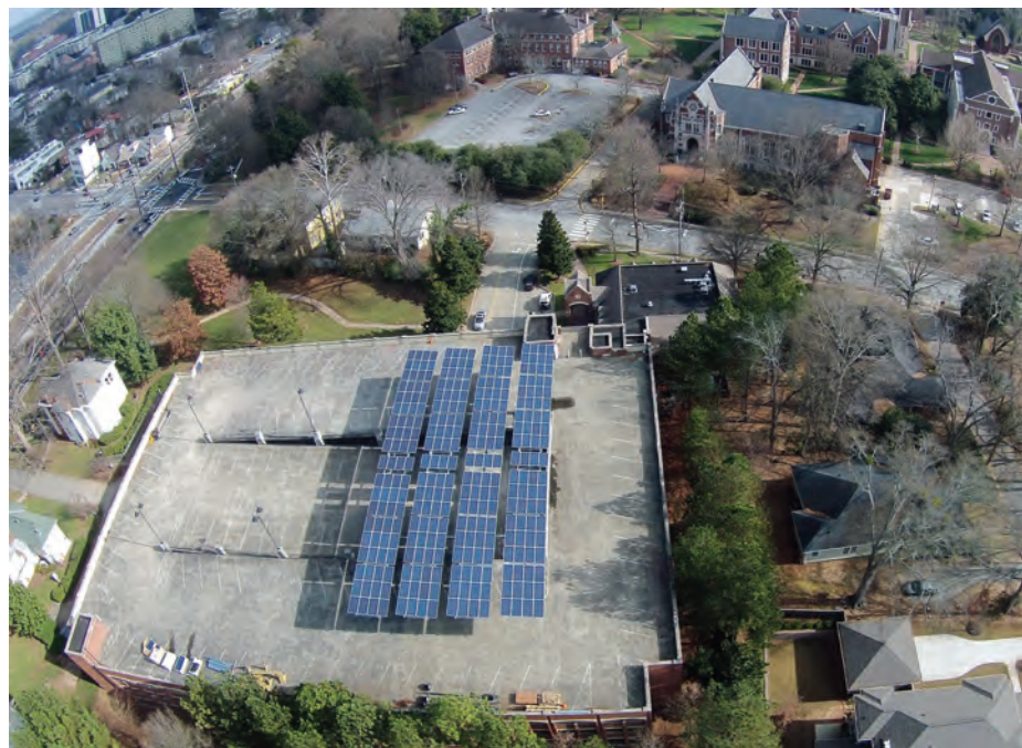
Centrally located on campus, the West Parking array is easily accessible to the college community and visitors. Photo courtesy Inman Solar.
