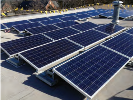
Ballast-mounted solar PV panels, like those installed on Bullock Science Center (above), use concrete to hold the array to the roof. This mounting option reduces the potential for roof damage. Photo courtesy Inman Solar.
