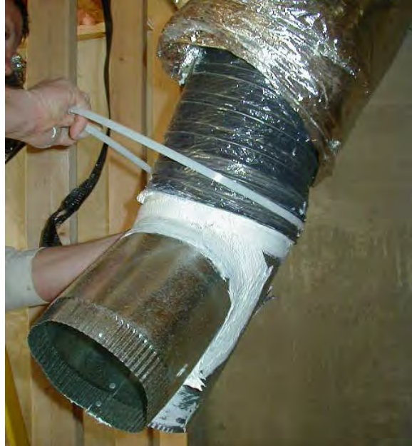
CORRECT: Mastic-sealed Joints
