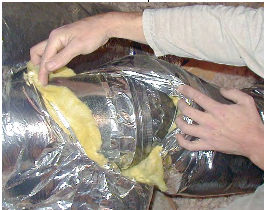
INCORRECT: UL-181 Tape without Mastic
