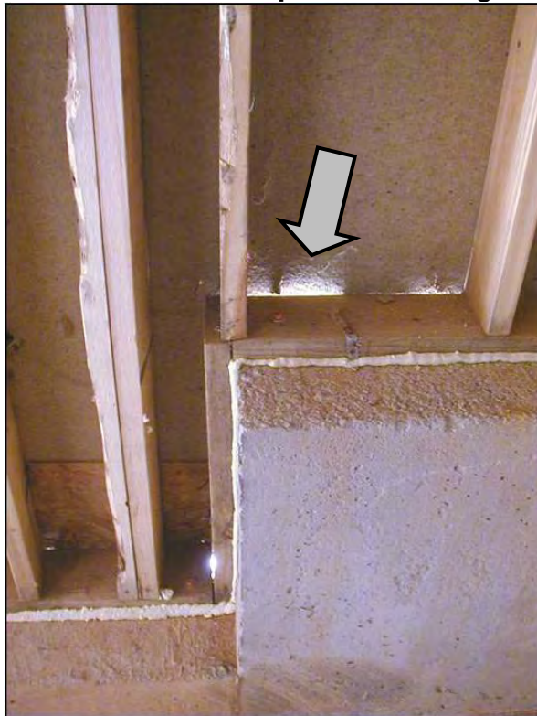
INCORRECT: Gaps in Sheathing
