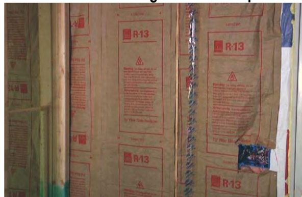
CORRECT: Full Coverage and No Compression
