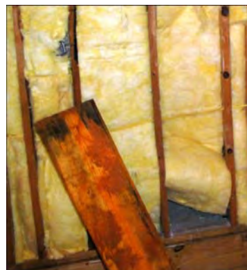
INCORRECT: Unfilled Cavity
