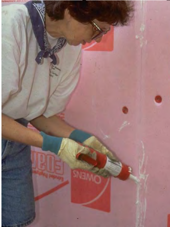
CORRECT: Sealing Exterior Sheathing
