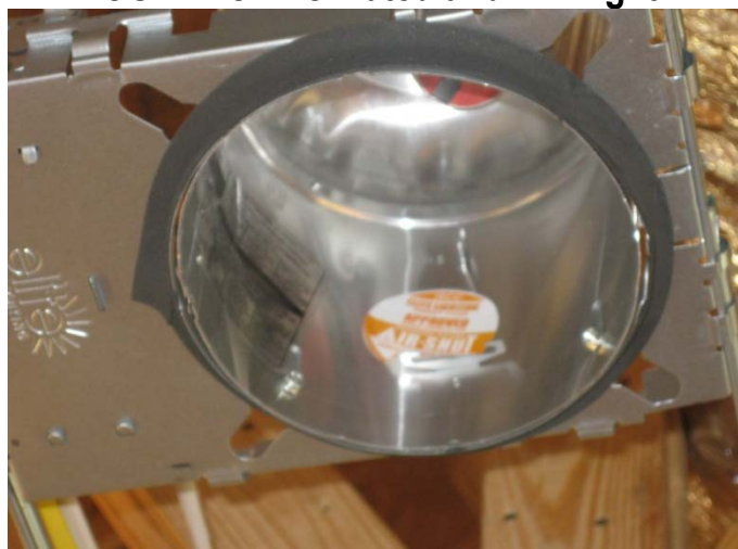
CORRECT: IC-Rated and Air-Tight
