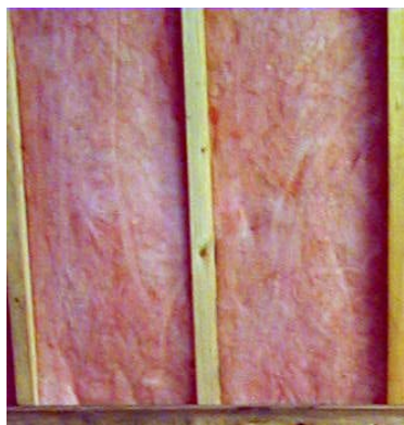
CORRECT: Batt in Wood-framed Cavity
