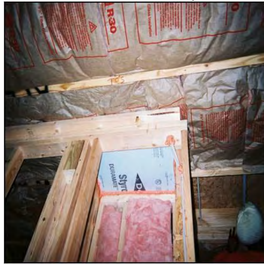
CORRECT: Well-sealed Chase (Prior to Duct Installation)
