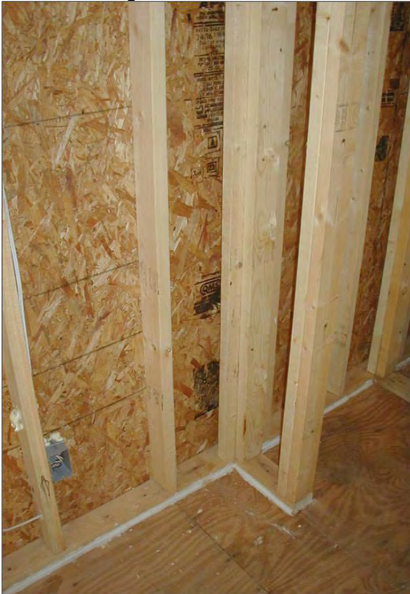
Caulking Around Bottom Plate
