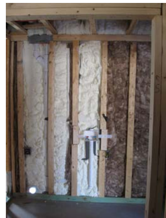
The laundry room wall of this new Chatham County home is sealed with fiberglass batt and spray foam insulation.
