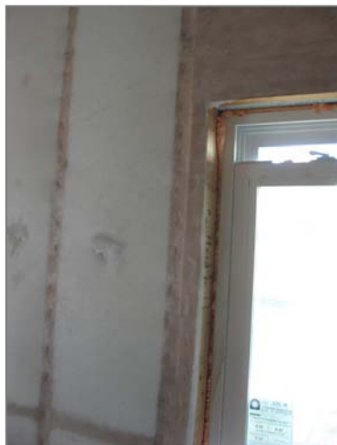
Blown-in cellulose is inspected during the insulation inspection of a multifamily building in Savannah. The NFRC sticker and air sealing around the window were inspected.
