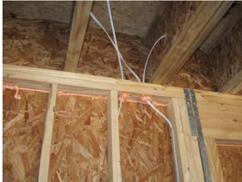
Sealing of framing and wall top plate can be seen on a new home under construction in Chatham County.
