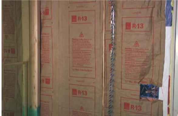
**INCORRECT: Compression and Poor Coverage**
