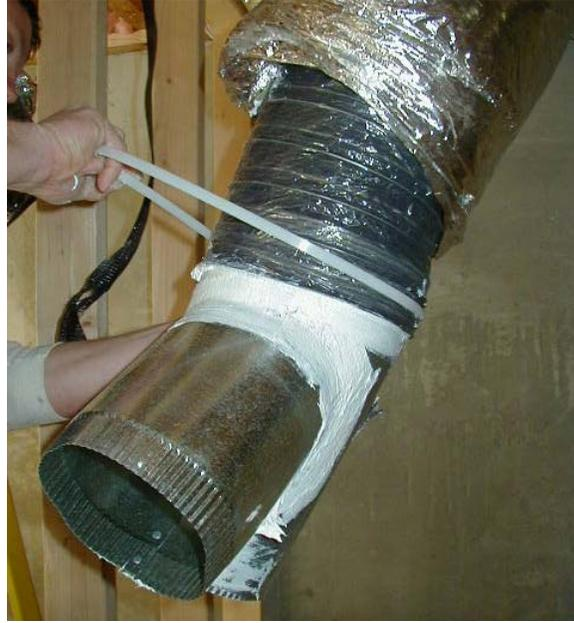
**Duct Sealing Diagram**
