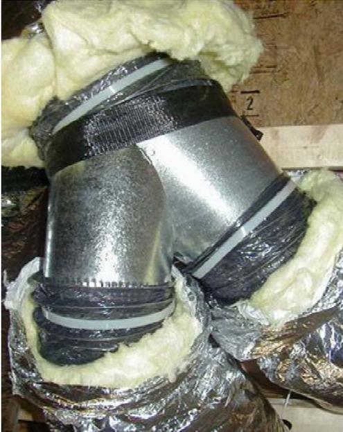
**CORRECT: Mastic-sealed Joints**
