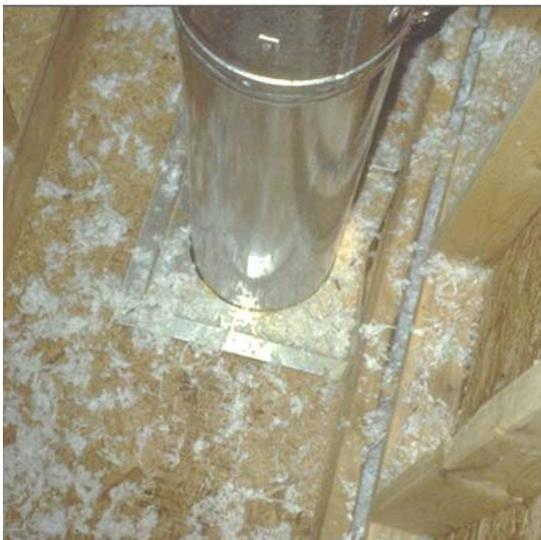
**CORRECT: Well-sealed Chase (Prior to Duct Installation)**
