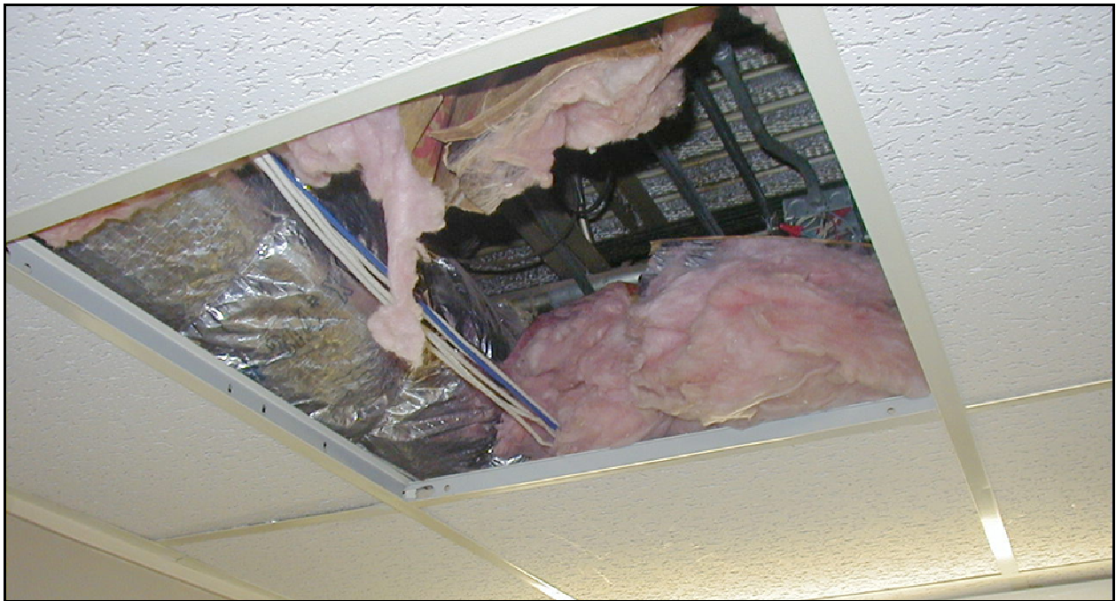
Envelope insulation may not be installed on top of suspended ceiling panels.
